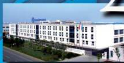
Marposs plant in China
